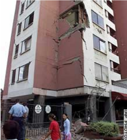
Figure 1. Residents stand outside a damaged building in Cali, Colombia (Photo courtesy of AP)
