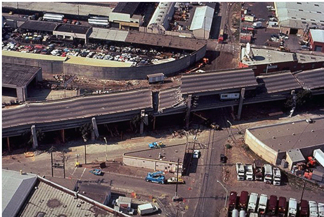
Figure 4. Cypress Viaduct Failure
