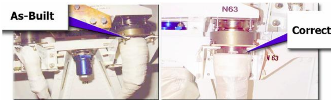
Figure 11-5. Electrical Harness as Built and Corrected
