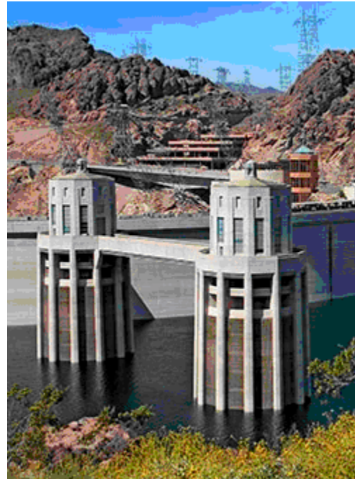
Figure 2. Two of the Four Intake Towers
