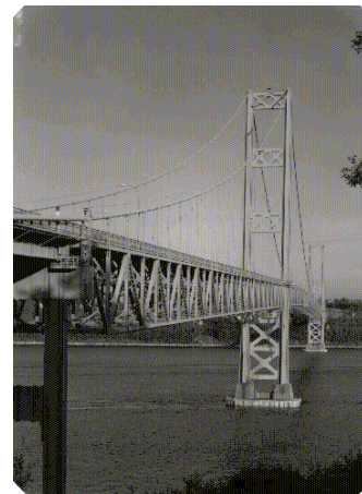
Figure 5. The Replacement Tacoma Narrows Bridge, Built in 1950
