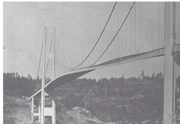
Figure 1. Torsional Mode of the Tacoma Narrows Bridge
