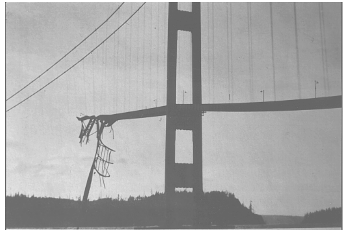
Figure 2b. Tacoma Narrows Bridge after the Failure
