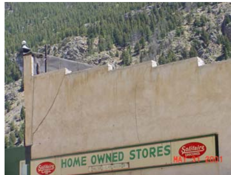
Figure 3. Condition of monitored structures.
