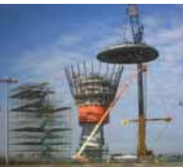
13. Locating cab roof onto 24 mullions.
