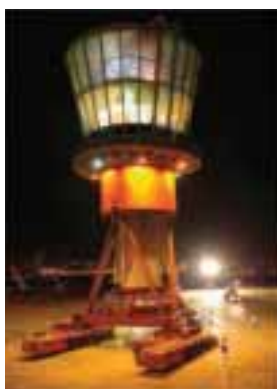
14. Moving 900 tonnes 1.5km across the airport.
