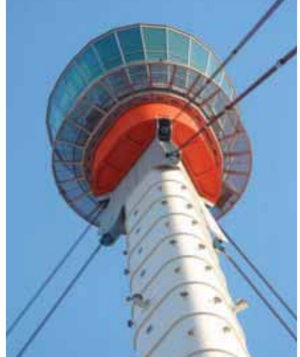
3. The 10m high glass façade provides a large cone of vision.
