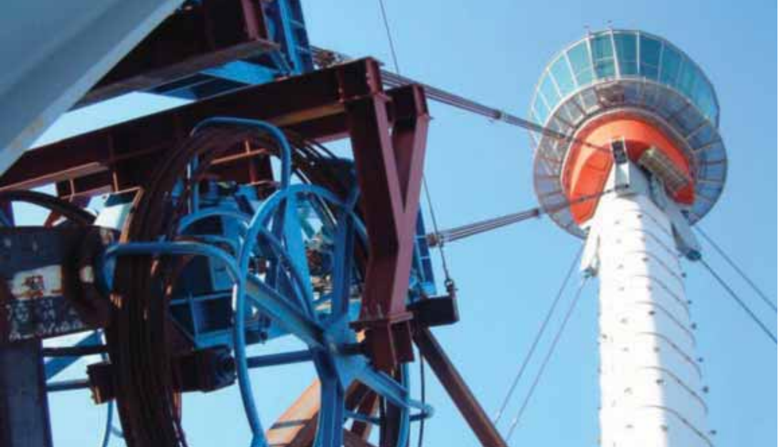
16. Jacks controlling guy cables during the lift.
