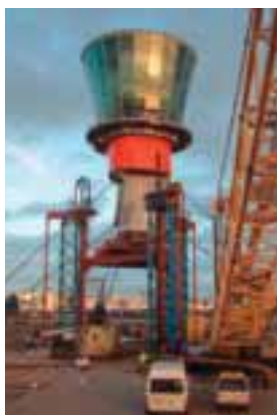
15. Jacking the cab to 87m height.
