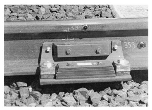
Figure 3. Rail vibration absorber attached to 115 lb/yd RE rail at the Portland Tri-Met ballast-and-concrete-tie track.
