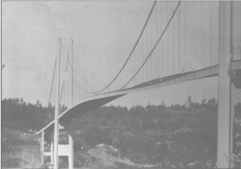
Figure 23.1. Torsional Mode of the Tacoma Narrows Bridge
