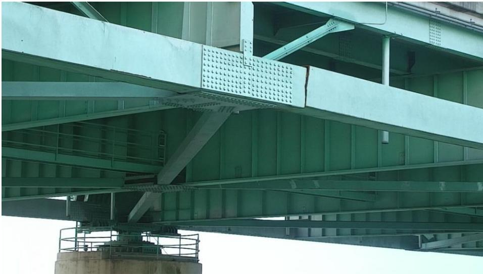
Figure 4.6. Interstate 40 Bridge Crack
