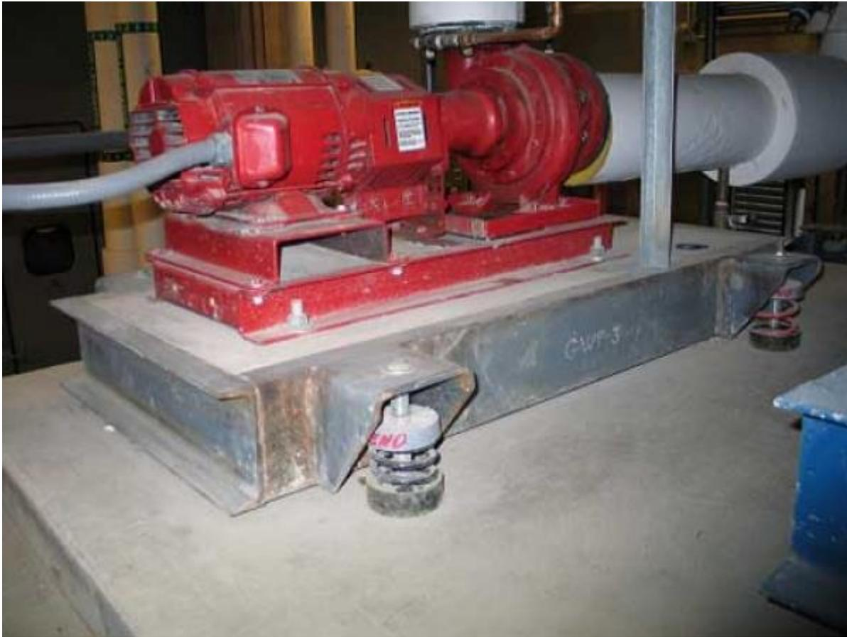
Figure 17.8. Pump Mounted to Floor via Inertial Frame & Springs
