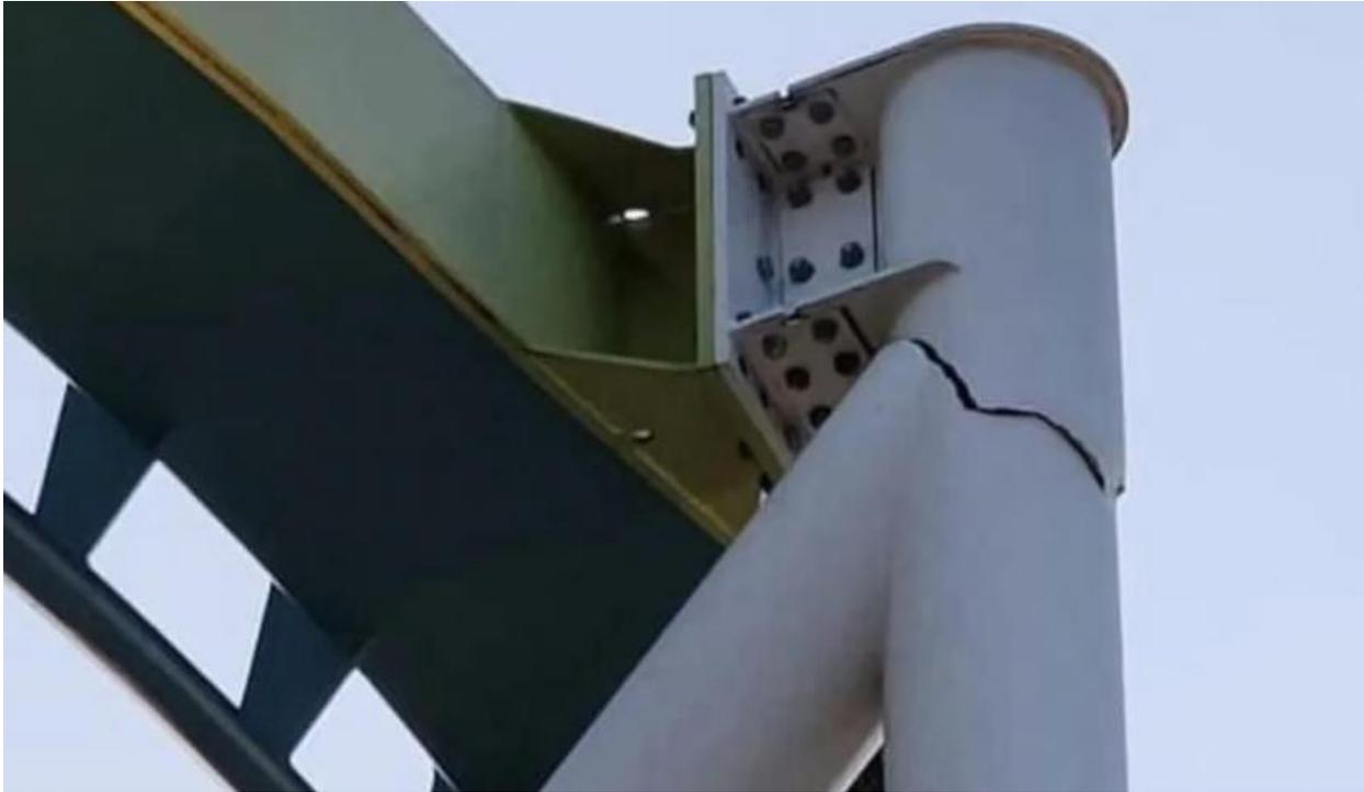
Figure 4.7. Roller Coaster Pillar Crack
