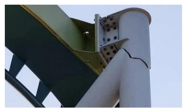
Figure 4.7. Roller Coaster Pillar Crack
