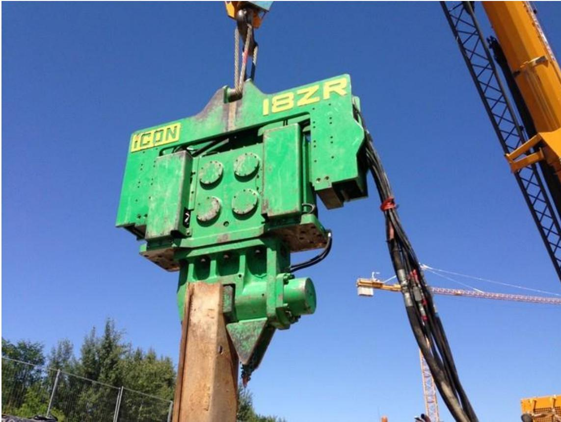
Figure 18.4. Vibratory Hammer Suspended from Crane Boom for Pile Driving
