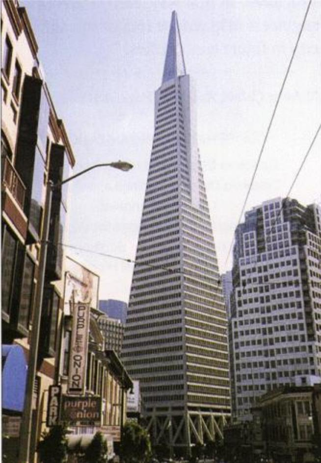
The Transamerica Pyramid is built from a steel frame, with a truss system at the base. The height is 850 ft (260 m). Reference [19] gives natural frequency and damping as obtained in the 1989 Loma Prieta earthquake and from ambient vibration. The ambient vibration was presumably due to wind, low-level micro-tremors, mechanical equipment, outside street traffic, etc.
