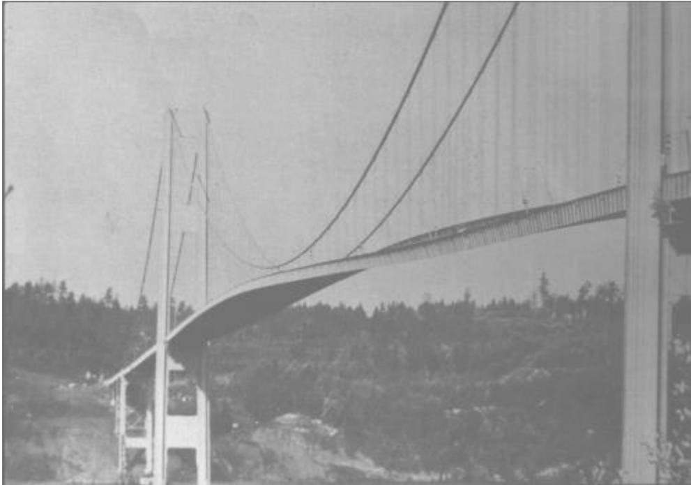
Figure 7.1. Torsional Mode of the Tacoma Narrows Bridge
