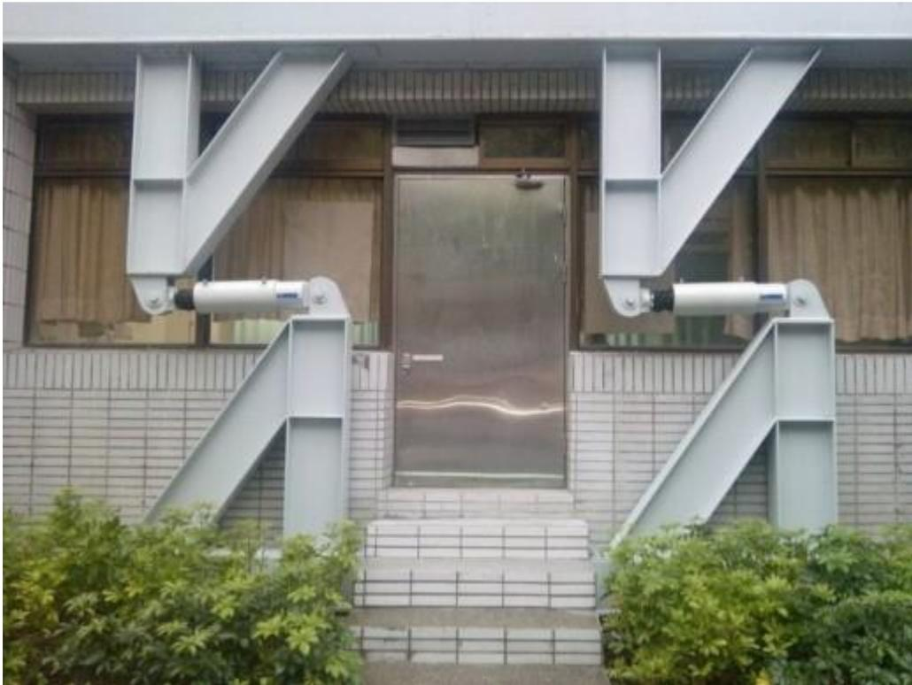
Figure 15.2. Shock Absorber for Seismic Isolation of Taipei City Hospital
