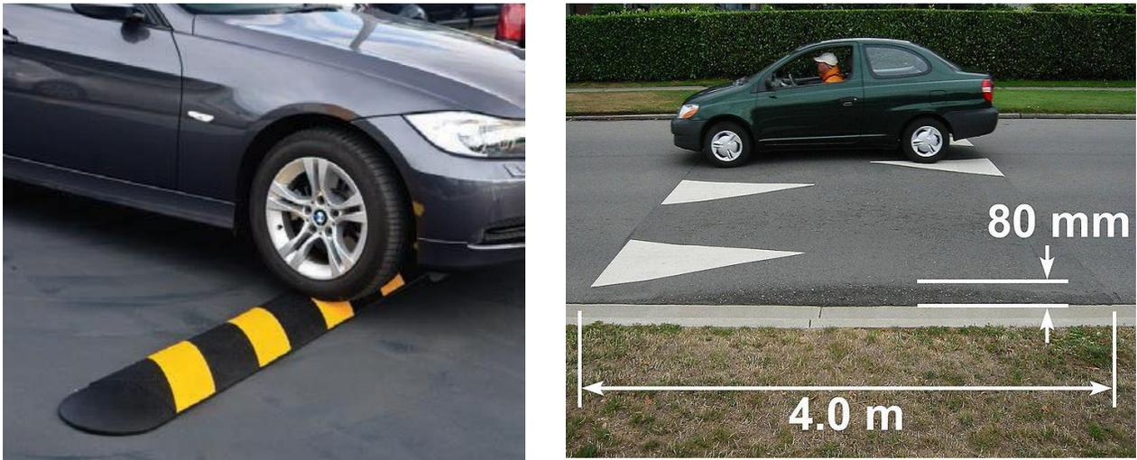
Figure 6.5. Speed Bump (left) and Hump (Right)
