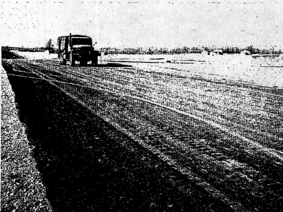
Figure 14. High speed paved road.
