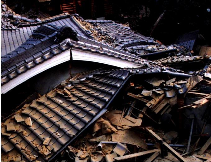
Fig. 3: Collapse of old timber house with heavy roof
