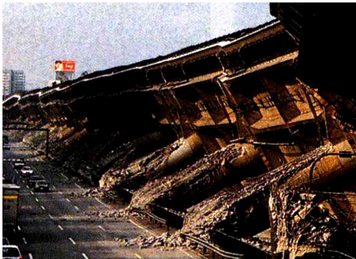
Fig. 1: Collapse of highway overpass
