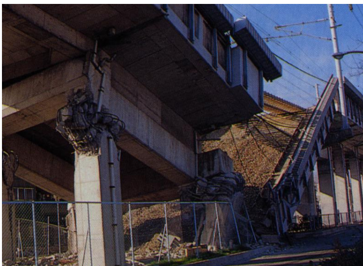
Fig. 2: Collapse of the Shinkansen overpass
