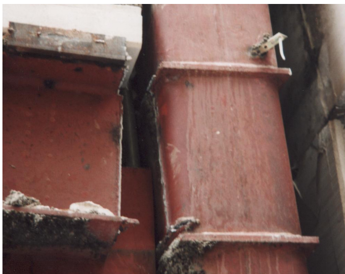
Fig. 5: Failure of steel structure at welding connection
