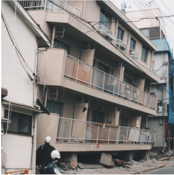
Fig. 12: Collapse of reinforced concrete buildings in first story
