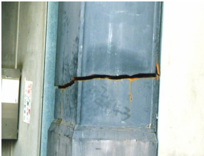
Fig. 6: Brittle fracture of large-size steel members
