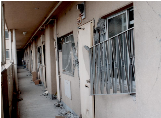
Fig. 14: Damage of non-structural elements
