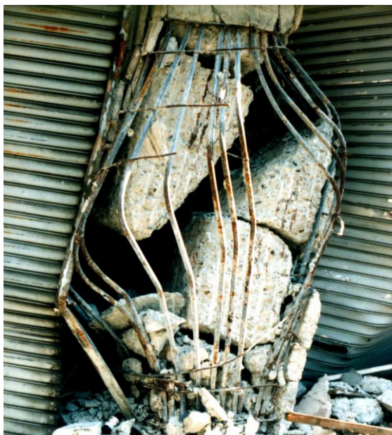
Fig. 8: Shear failure of reinforced concrete column
