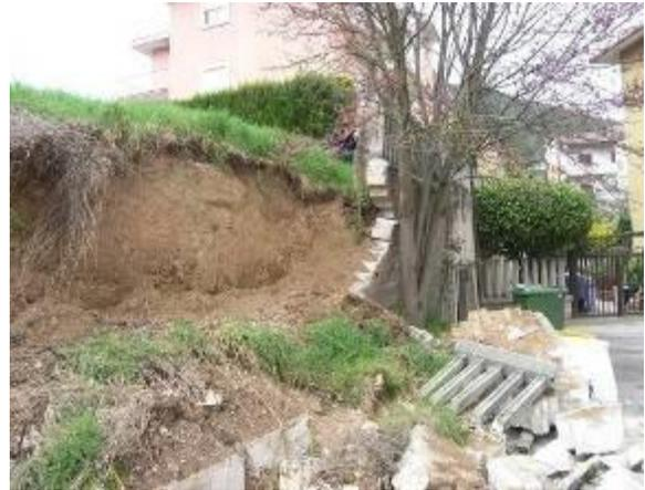
**Figure 11:** Total collapse of a wall from the L'Aquila earthquake (GEER).
