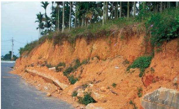
**Figure 13:** This wall sank into the earth due to insufficient pressure support at its toe (Fang 1148).
