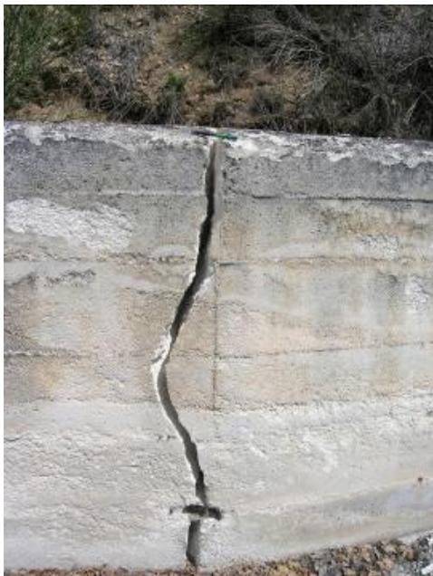
**Figure 10:** Cracks due to the L'Aquila earthquake (GEER).
