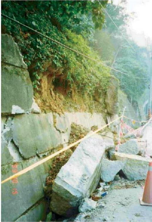
**Figure 12:** This retaining wall was not reinforced; it failed at the mortar joints (Fang 1144).
