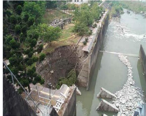
**Figure 14:** Shih-Kang dam spillway failure (USBR 2009).
