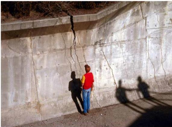
**Figure 15:** Loma Prieta: this retaining wall sustained major cracks (Wikipedia).
