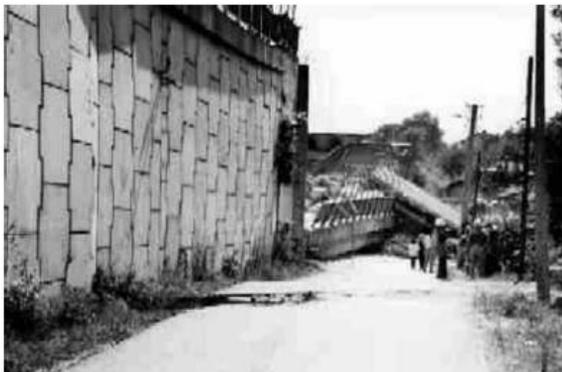
**Figure 20:** Reinforced earth wall after earthquake (Sankey 3).
