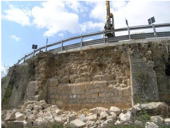
**Figure 9:** The masonry infill of this wall failed from the L'Aquila earthquake (GEER).
