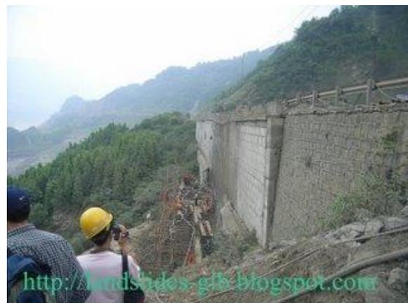
**Figure 19:** Embankment which had a small settlement at the middle.
