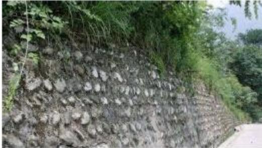
**Figure 16:** Stone and concrete retaining wall. (Source unknown).
