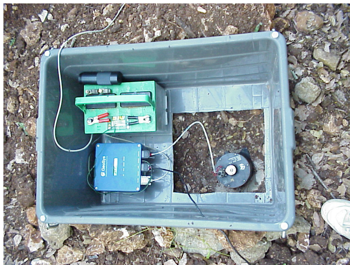
Figure 7.12 A simple field installation. A plastic box has been placed directly on the ground. The sensor is placed in the cut out hole. Inside is also the battery and recorder. The cable going out is for the GPS. After installation, soil was put up around the sides and insulation was put on top of the lid. The sensor is a Kinemetrics Ranger 1 Hz seismometer (Table 2.2) and the recorder a GeoSig GBV316 (Table 5.3).
