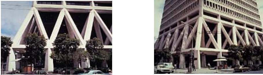
Figure 2. Truss System at Base of the Transamerica Building
