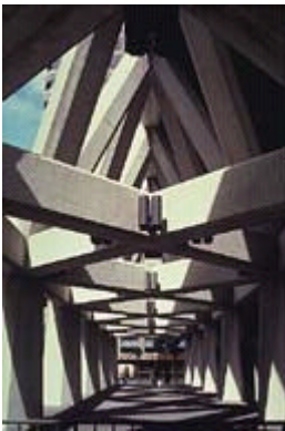
Figure 3. Horizontal X-bracing
