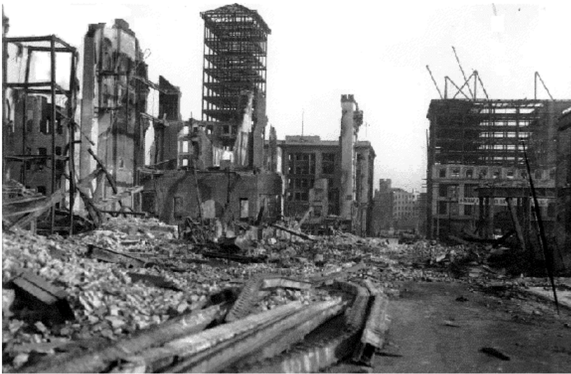
Damage at Union Square. Photo courtesy of the Museum of the City of San Francisco.
