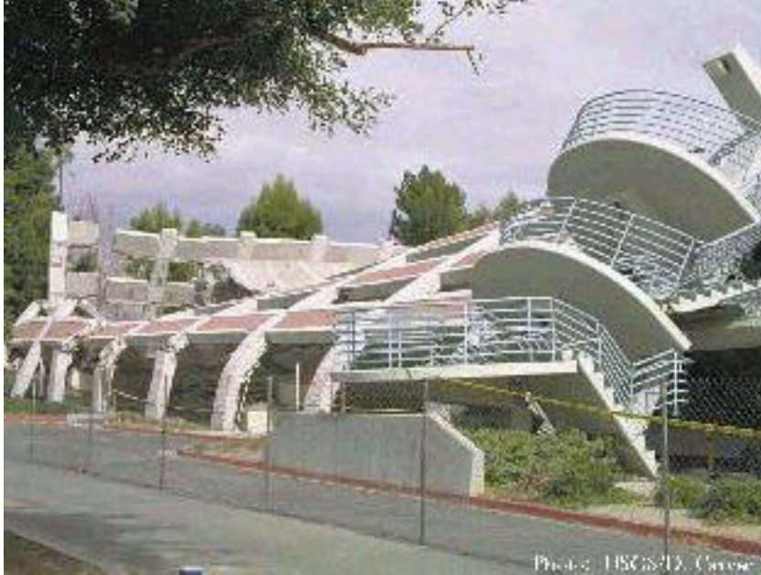
Collapsed Parking Structure, California State University at Northridge. Photo Courtesy of U.S. Geological Survey.
