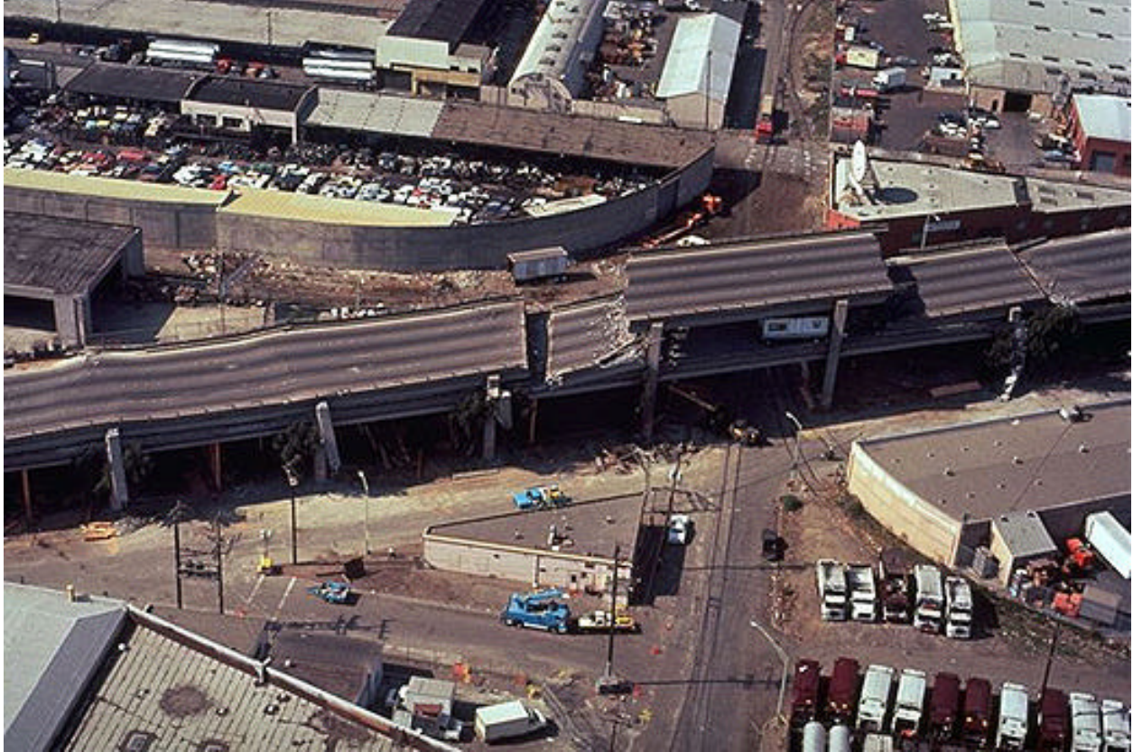
Collapse of Cypress Viaduct. Photo courtesy of U.S. Geological Survey.
