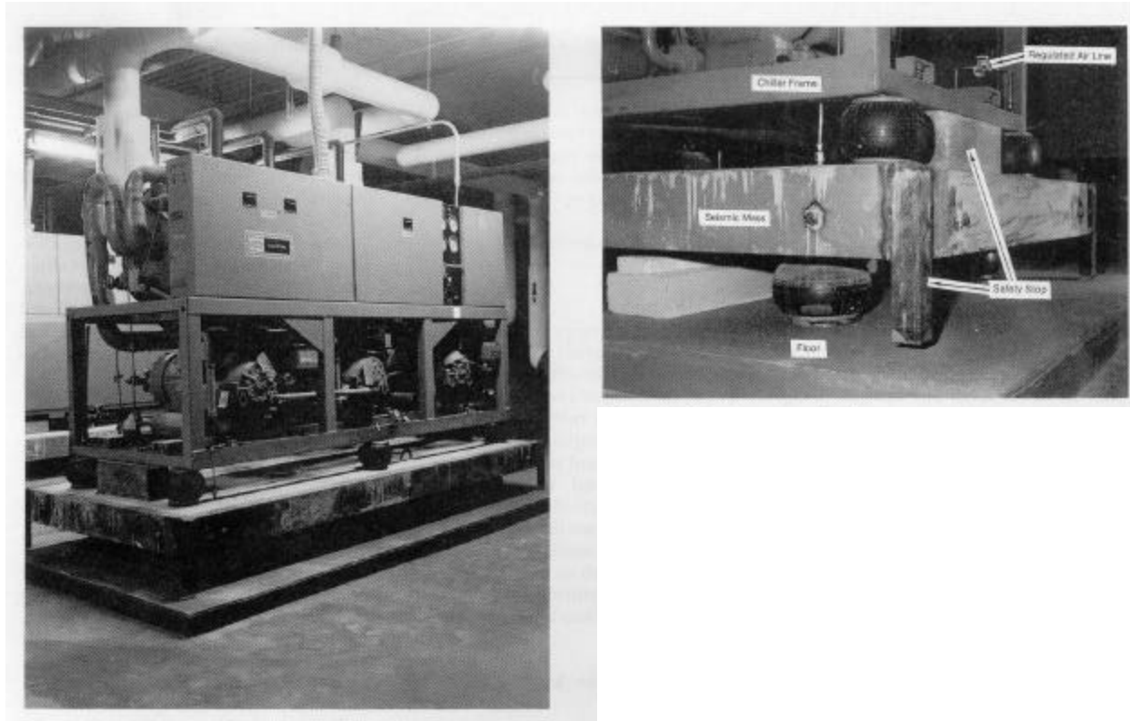
Figure 8. Air conditioner chiller installation, featuring a two level isolation system with a seismic mass (ref. Sound and Vibration, March 1985)
